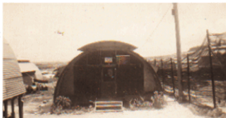
Here is the exterior of our "Lazy Lodge." Note the clothesline with the laundry between the two huts, the flowers in front, and the camouflage fence between the hospital and our hut.
